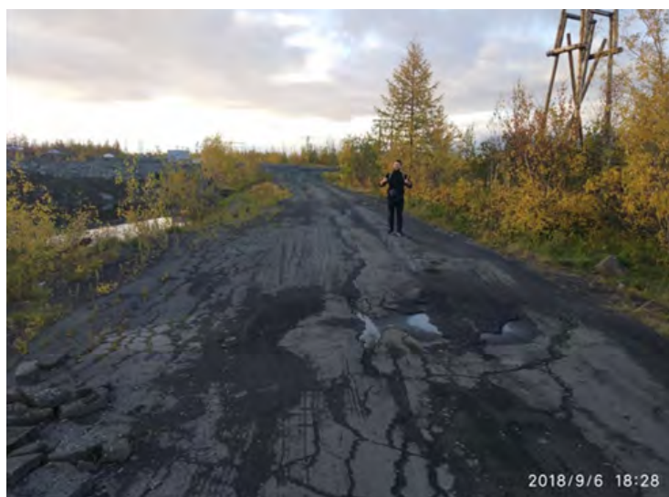
Fig. 3. Deformation of the road surface as a result of the development of thermokarst and the melting of polygonal ice under the road embankment (photo by Tolmanov V.A., September 2018).
